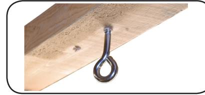
2. The ceiling mounting bolts must be attached to wall studs or ceiling rafters. If the studs or rafters are covered by drywall, use a stud locator to find. Using the distance calculated in the step above, mark the two hole locations. Using a 3/32" bit, drill pilot holes and screw the bolts inward until no threads are showing
